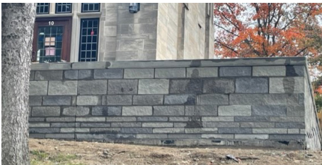
Refectory terrace construction as of 10.20.2022
