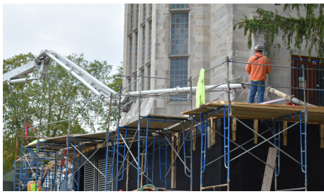
Refectory terrace construction as of 10.06.22
