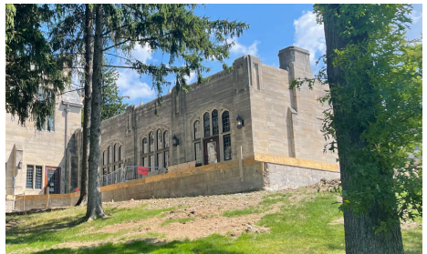
Refectory terrace construction as of 8.23.22.
