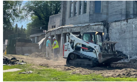
Refectory terrace construction 7.18.22.
