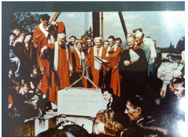
9/23/1951 Laying of the Cornerstone - historical files
